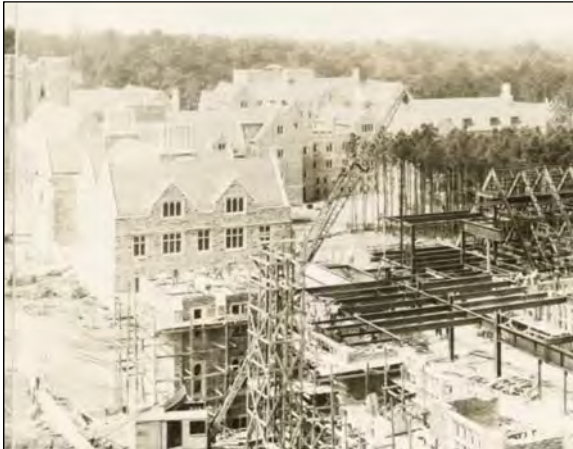
Duke University, West Campus construction, August 1930
