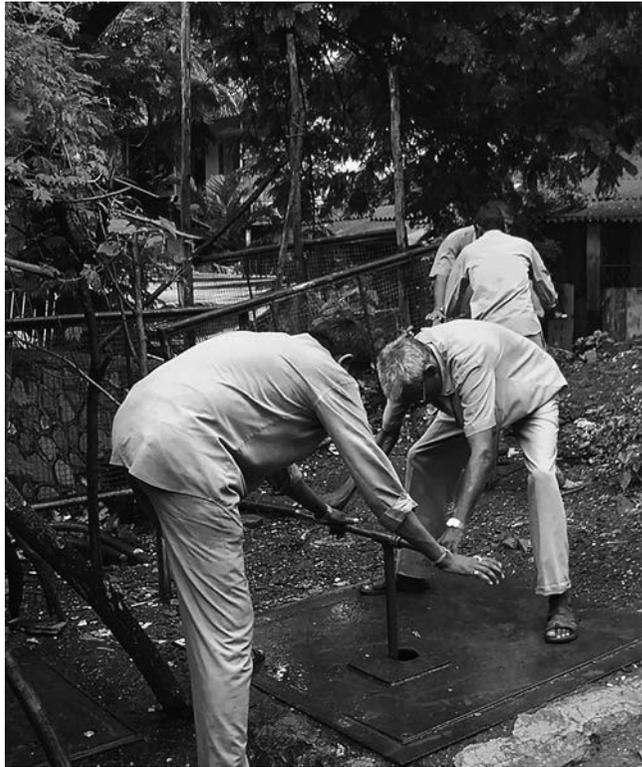
because the amount of water the city gets every day is finite and materialized by valve operations, to give one hydraulic zone more water is also to give another zone less.
