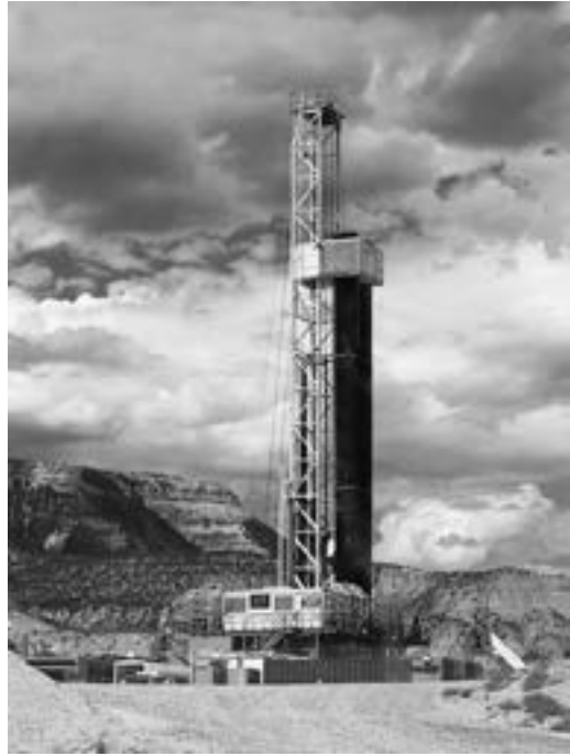
FIGURE I.5. Flex rig for directional drilling. Photo by the author.
